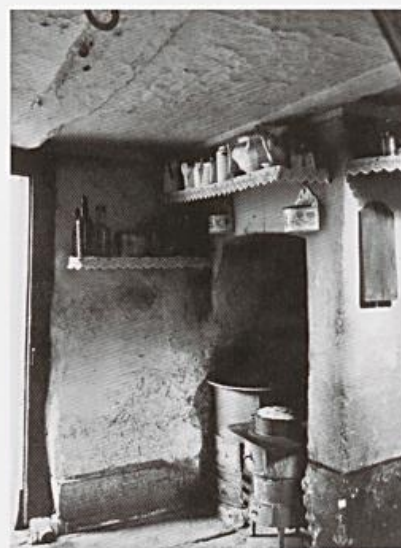
Formerly open hearth with an iron stove and mantled oven placed in the chimney casing, Detmold, Auguststrasse 11, um 1900
