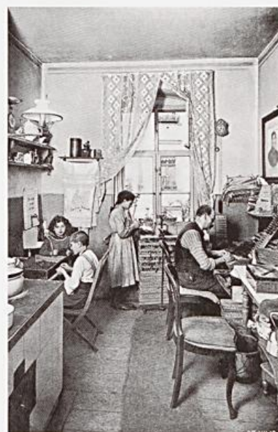
1858 Kitchen of outworkers in a Berlin tenement, 1910, With tiled hearth, gas lighting and faucet with sink
